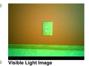
**IR000150.IS2** 3/19/2009 1:50:33 PM Air leak detected on electrical outlet on exterior wall in kitchen. Recommend air sealing with foam, caulk or foam gasket.
