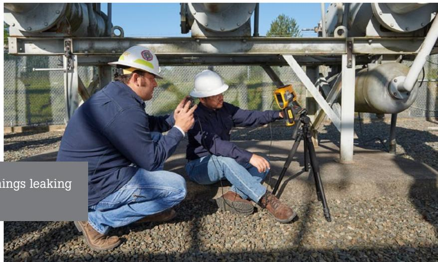
“With the camera, you can see things leaking before there is a pressure loss,”
