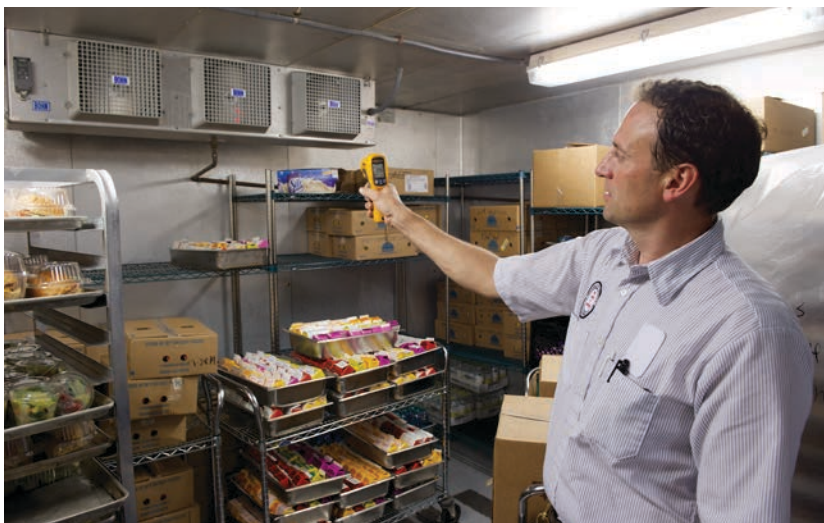
Mark uses his 62 MAX Infrared Thermometer to check refrigeration units in a walk-in cooler, as part of his preventive maintenance program.
