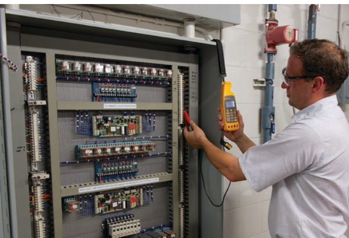
With his Fluke 773 Milliamp Process Meter, Mark checks the control signal loop in the low-voltage relay cabinet.
