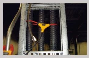
Linamar technicians clamped the iFlex<sup>™</sup> flexible current probe around the three feeder cables at each compressor to measure phase current unbalances. Photo courtesy of Linamar Corporation
