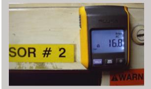
The Fluke 381 clamp meter's remote display attached to compressor #2 provided easy monitoring from several feet away. Photo courtesy of Linamar Corporation
