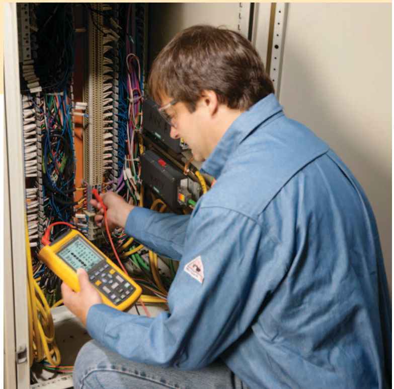
Figure 1. Effective troubleshooting may require an examination of wiring, connections, and the electrical characteristics of signals as they traverse the system.
