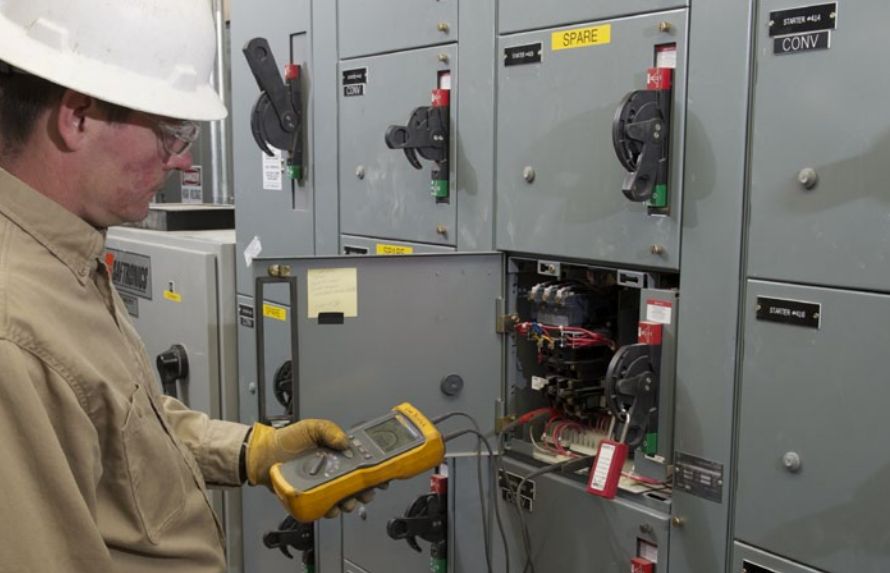
These modern panels are part of Keithly's system redesign for a client. Here Greg Burdick uses a Fluke 1520 megohm meter to test insulation on an out-of-service circuit.
