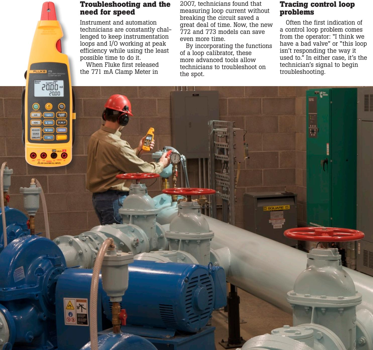
The first step is to measure the 4-20 mA signal, either by breaking the loop connecting in series with a DMM, or by using a mA clamp meter like the Fluke 771 and verifying the loop current value. If the loop current measured is not as expected, there are three likely causes: broken/disconnected/shorted wires, a bad loop power supply, or faulty instrumentation.
