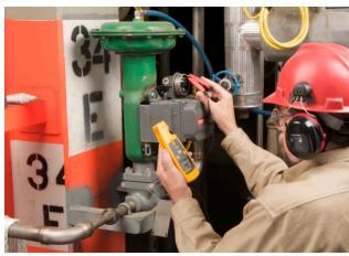
Checking a Fieldvue control on a Fischer valve for a condensate collection system.
