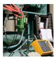
Many HVAC techs are finding that logging power usage of HVAC systems gives them the data they need to convince clients to upgrade to new, more efficient systems. This tech is using the Fluke 1735 Power Logger.
